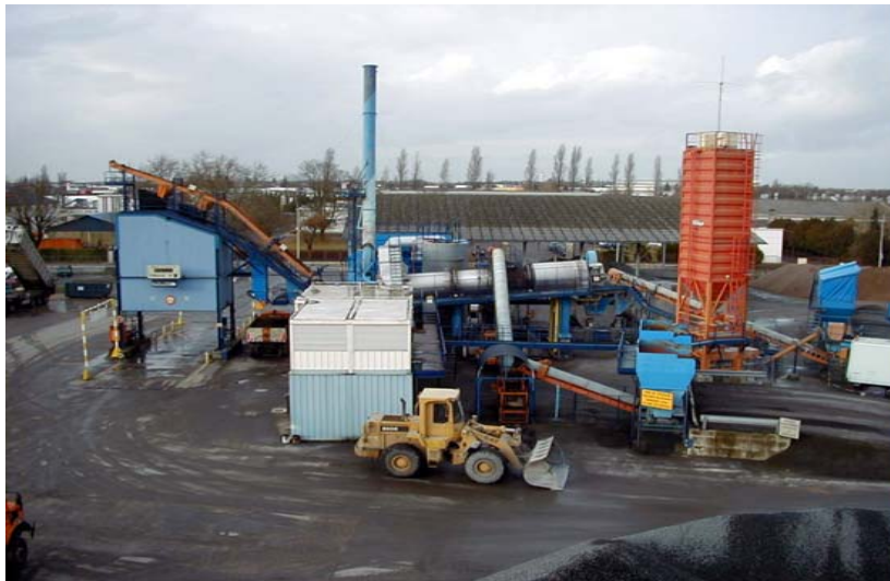
Production site (Drum mix plant)
